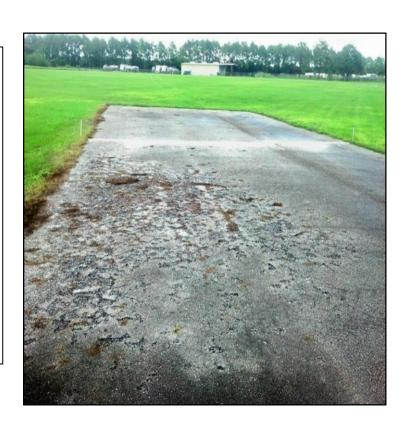
The proposed repairs would include filling many of the larger cracks and repairing the area on the pylon staging runway with hot asphalt. Several of the larger damaged areas on the concrete taxiways were also filled.
