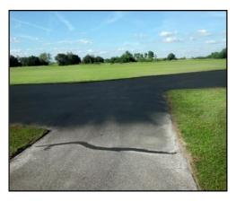
The rains and weather the earlier part of the month slowed the process down a little but eventually all of the prep work was completed and after a final cleaning with a heavy duty blower, the process was underway! First, the main runway was sealed. This took two applications as according to Capt. Mike Porter the asphalt just seemed to suck-up the first coat.
